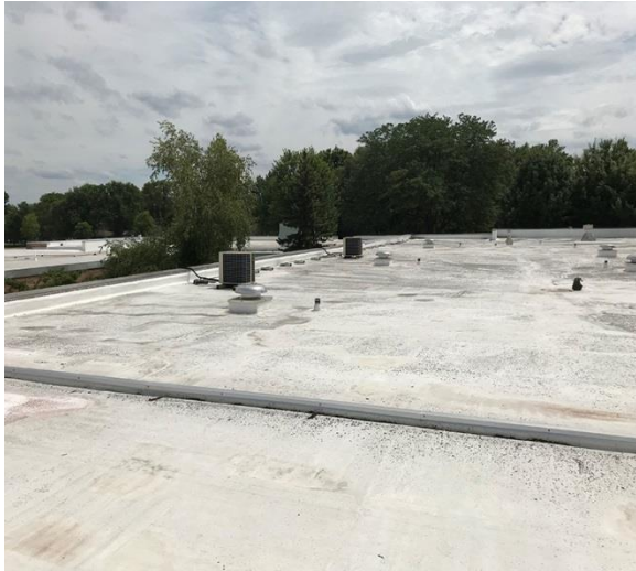
TPO Roofing with Scrim Showing
