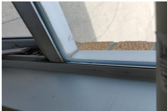
Single Pane Glazing at Original Building Classrooms
