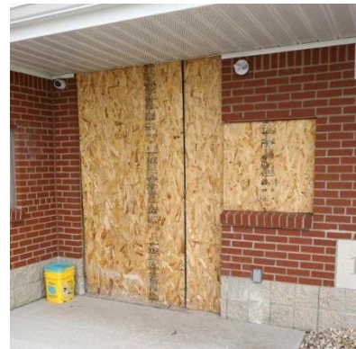
Construction Near Main Entrance
