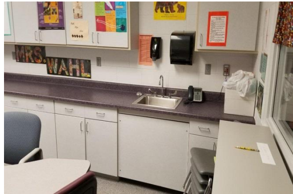
Casework in Administration Area With Removable Panel Under Sink
