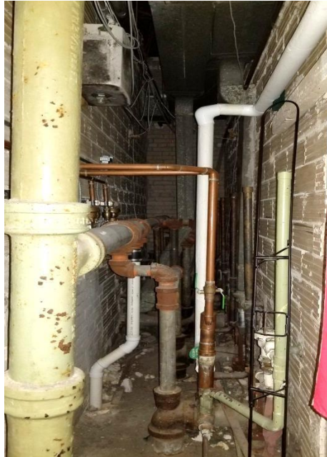
Plumbing at Chase
