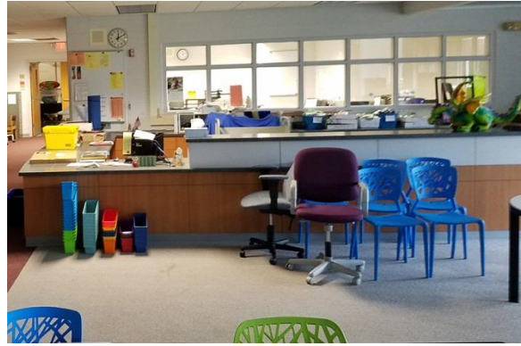
ADA-Required Transaction Height at IMC Casework
