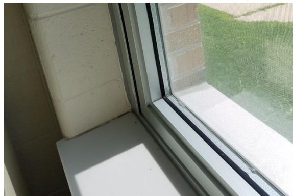
Insulated Glazing at Addition Classrooms
