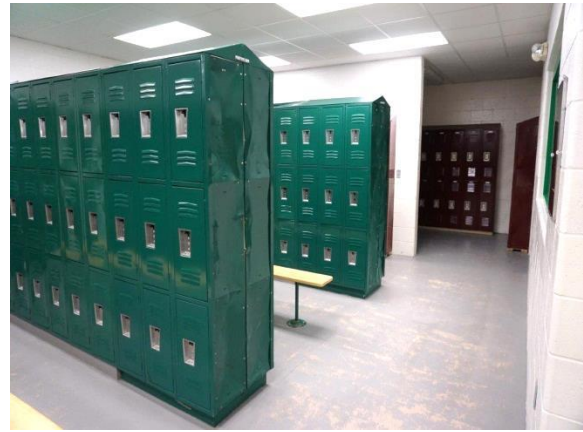
Damaged Lockers and Non-ADA Compliant Bench
