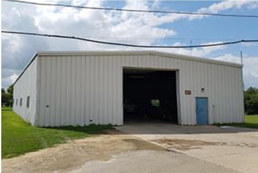
Exterior Metal Storage Shed
