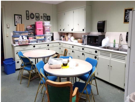
Non-ADA Compliant Casework/Sink at Break Room
