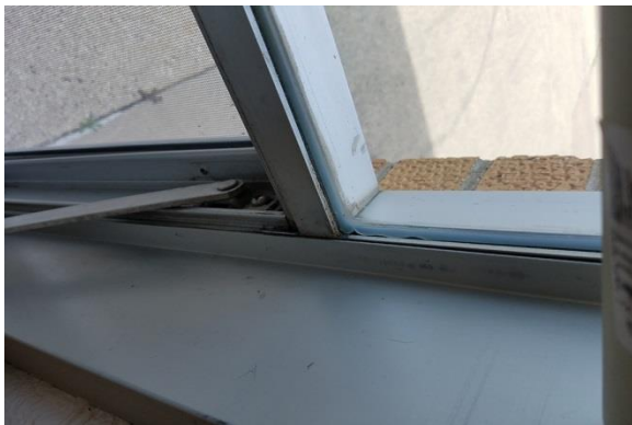
Single Pane Glazing at Original Building Classrooms
