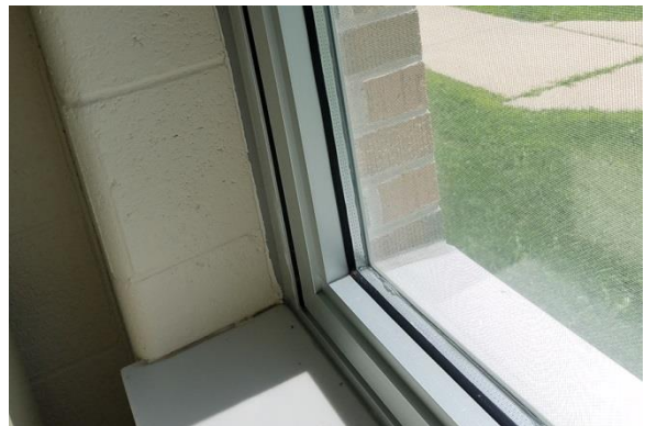
Insulated Glazing at Addition Classrooms
