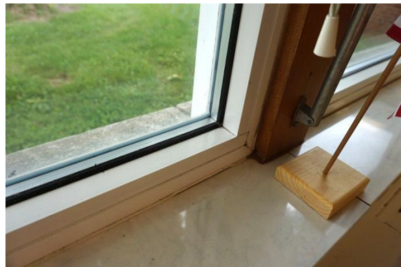
Insulated Glazing at Addition Classrooms
