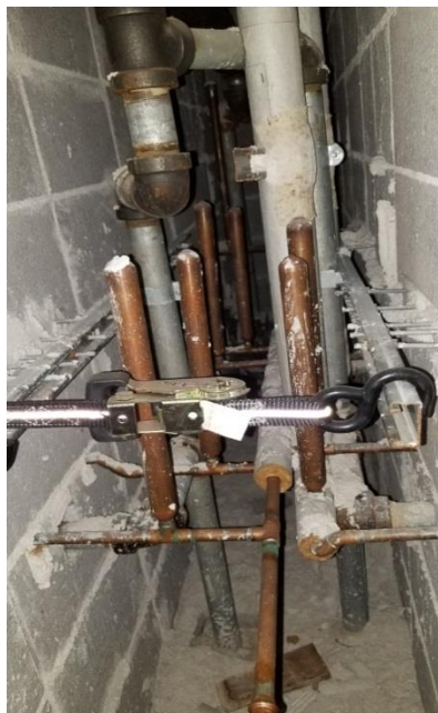
Plumbing Chase at Toilet Rooms
