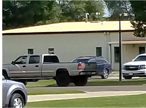
Existing PVC Roof Membrane
