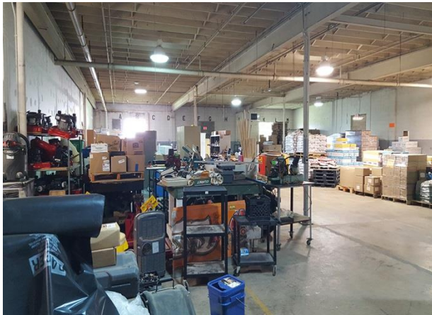
Uninsulated Storage/Maintenance Area
