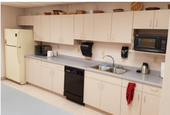
Non-ADA Compliant Counters/Fixtures at Staff Room
