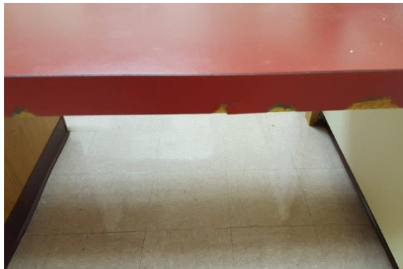
Damaged Countertop Edges
