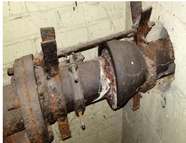
Sanitary Piping Connection
