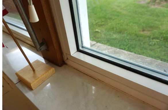
Single Pane Glazing at Original Building Classrooms
