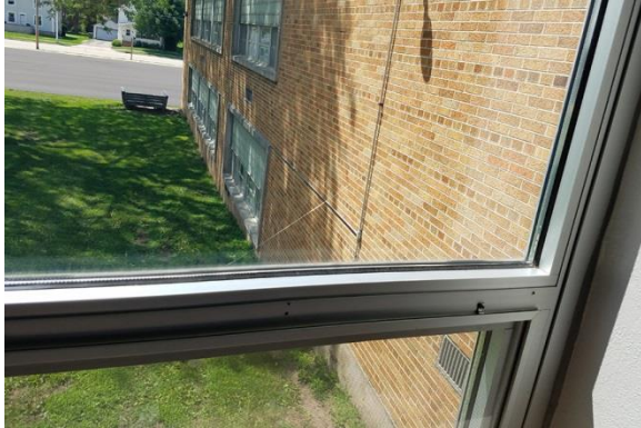
Insulated Glazing at Addition Classrooms
