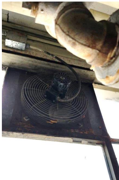
Single Pane Window, Ventilation Fan
