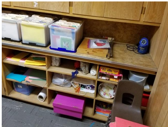
Older Wood Casework at Classroom
