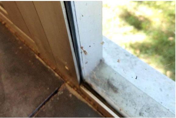
Single Pane Glazing at Original Building Classrooms
