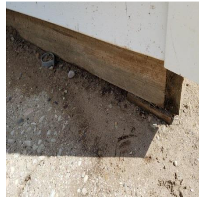
Wood Framing for Foundation
