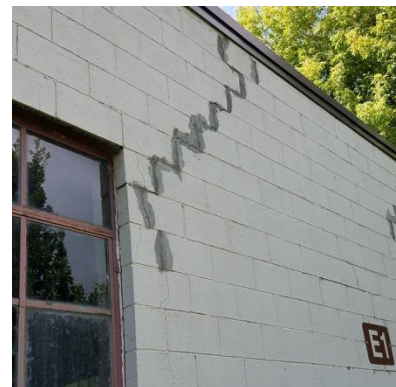
Previous CMU Repair
