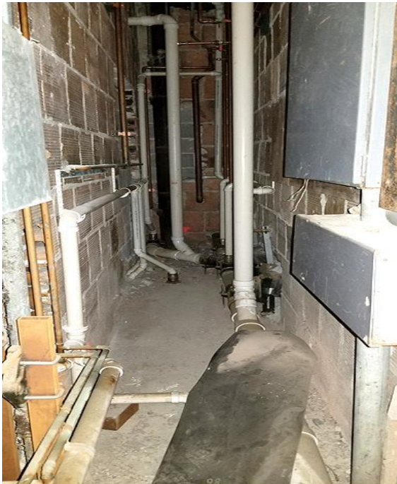
Pipe Chase with Renovated Piping
