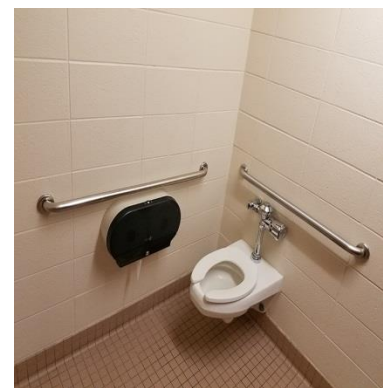
Missing Grab Bars at ADA Toilet Room
