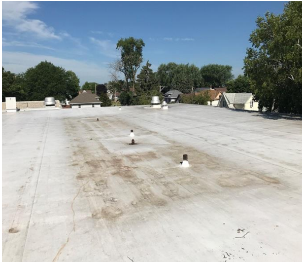
TPO Roofing with Scrim Showing
