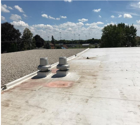
Existing Ballasted and Fully Adhered Membrane Roof
