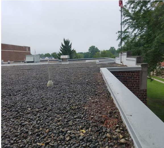
Existing Ballasted TPO Roof
