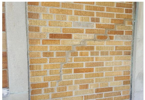
Previous Masonry Repairs
