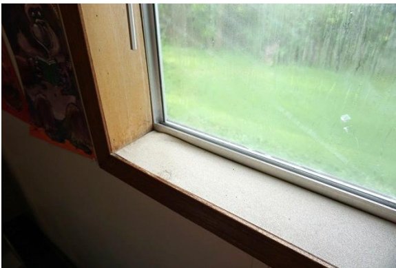
Single Pane Glazing at Original Building Classrooms
