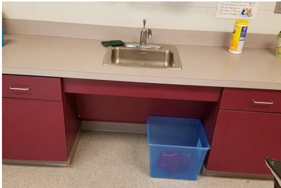
ADA Required Knee Space at Classroom Sink
