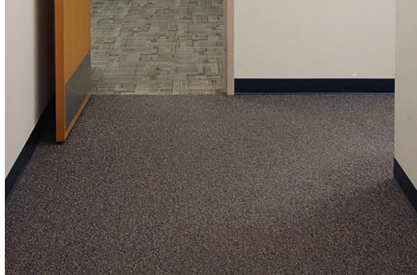
Carpet Transition at Corridor
