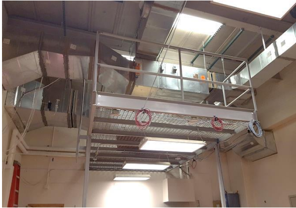
Mechanical Mezzanine Installed at Stage Area
