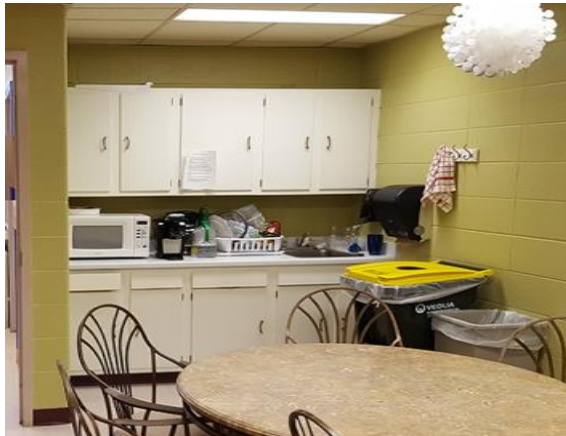
Non-ADA Compliant Casework at Break Room
