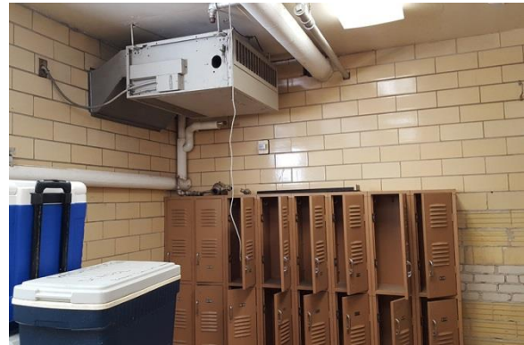
Abandoned Locker Room used as Storage
