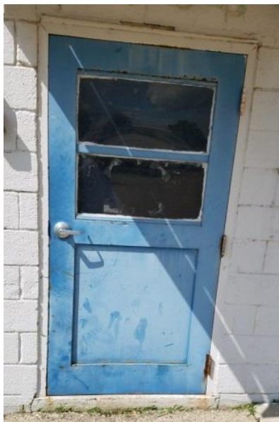
Original Exterior Wood Door
