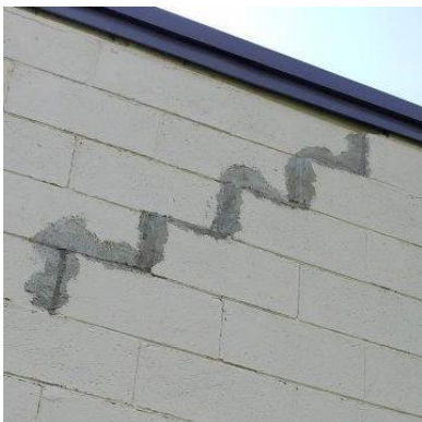
Previous CMU Repair
