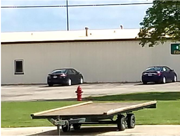
Existing PVC Roof Membrane
