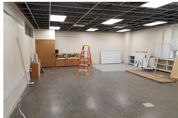
Classroom Under Renovation
