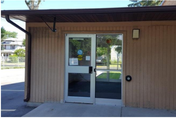
Vestibule Addition at W-1 Entrance
