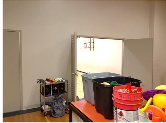
Infilled Stage Opening Facing Gymnasium
