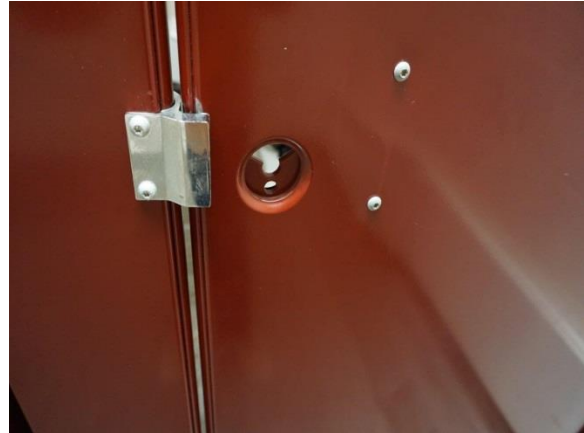
Missing Privacy Lock
