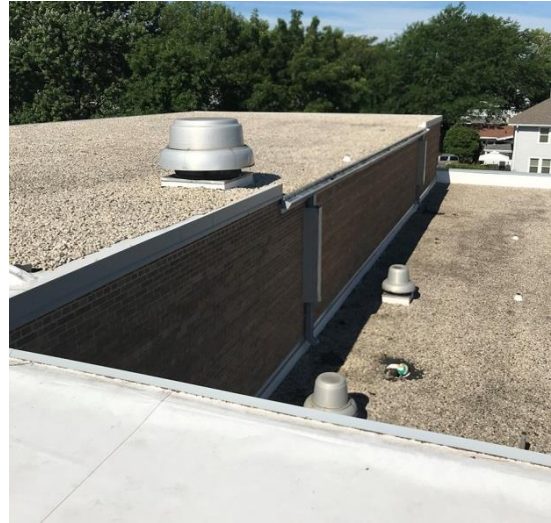
Existing Ballasted and Fully Adhered Membrane Roof
